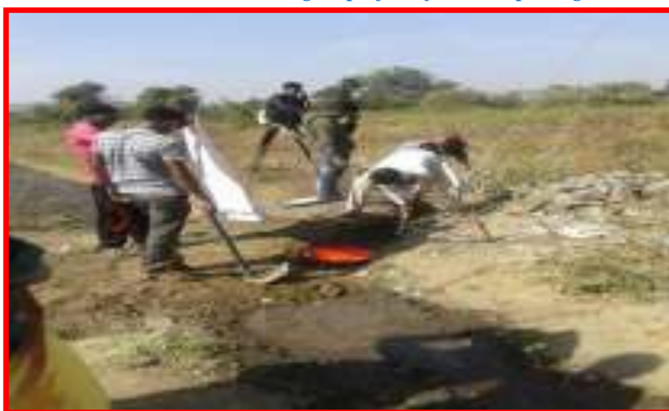
NSS Volunteer working on project of Digging Canal
