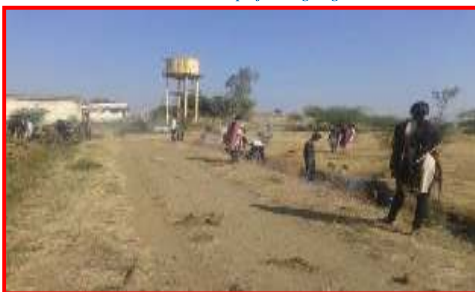
NSS Volunteer working on project of Road Repairing
